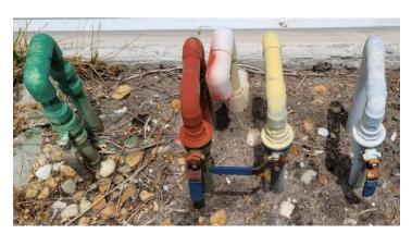
If the handle is in-line with the piping, the water is on to your unit; if the valve is 90 degrees from the piping, the water is turned off to your unit.
